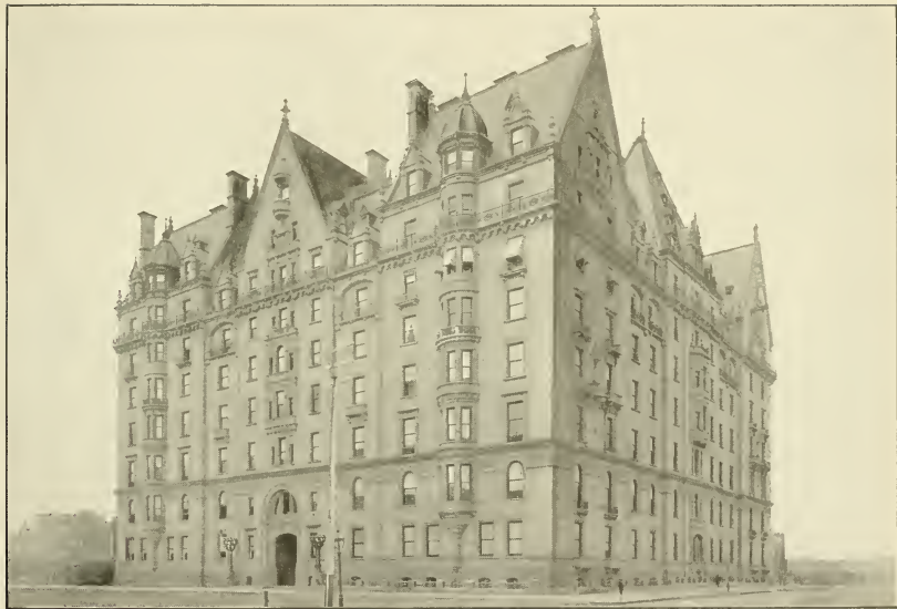
THE DAKOTA FLATS — Northwest Corner Central Park (West) and Seventy-second Street.
